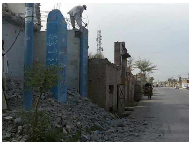
Photo 2: Removal of structures by the owners. December, 2015
