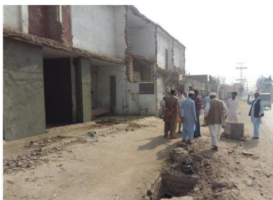
Photo 1: Structures repaired after voluntarily removing extended sections inside the ROW. Alizai Kaghawala: Chanaige 1224+000
