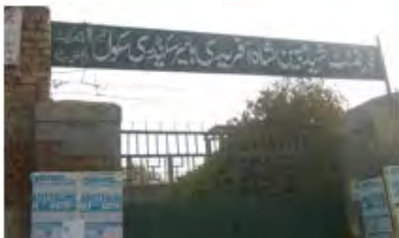
Photograph 11-11: Govt Shaheed Mobeen Shah Higher Secondary School
