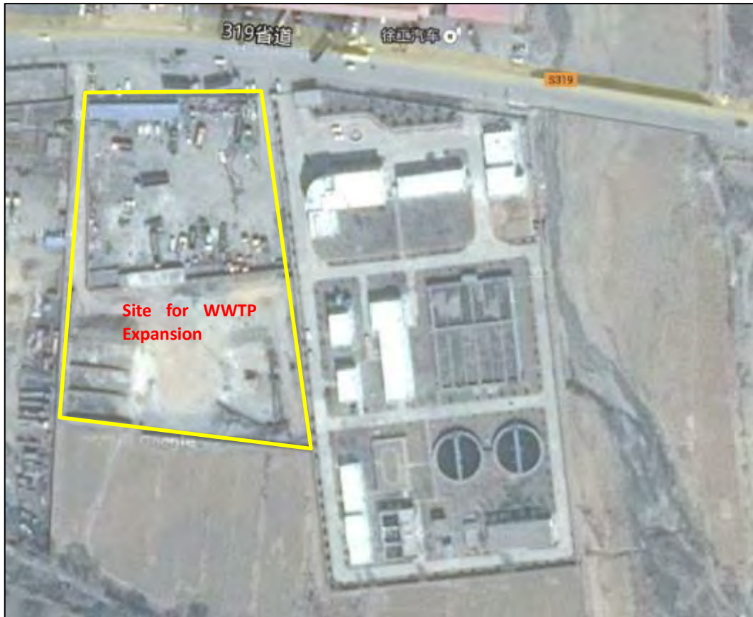
Figure IV-32. Satellite Photo of the Existing Zuoquan WWTP
