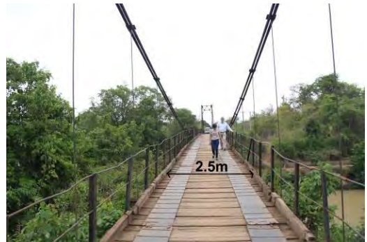
Ia Mor suspension bridge: 2.5m width
