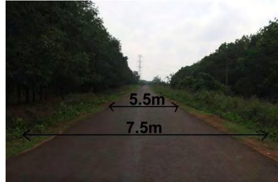
Bitumen section: 5.5m surface width – Rubber plantation area
