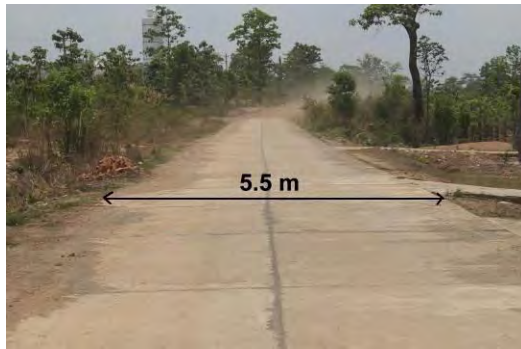
Cement concrete: 5.5m surface width
