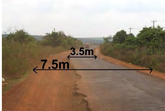
Bitumen section: 3.5m surface width
