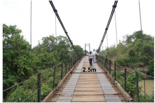
Ia Mor suspension bridge: 2.5m width
