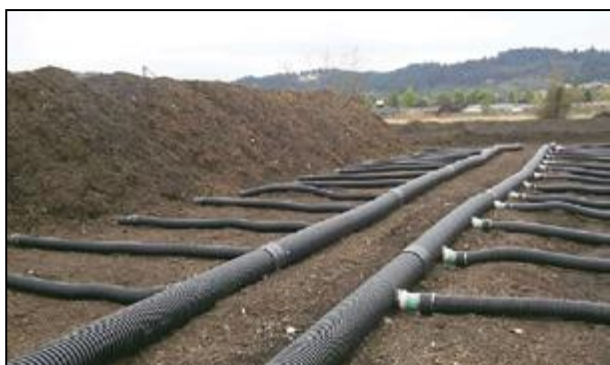
Figure 3-39: Example outdoor composting with aeration pipes system
