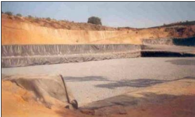
Figure 3-44: Liner system of Controlled Landfill
