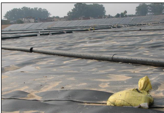
Figure 3-45: Leachate collection system of controlled Landfill
