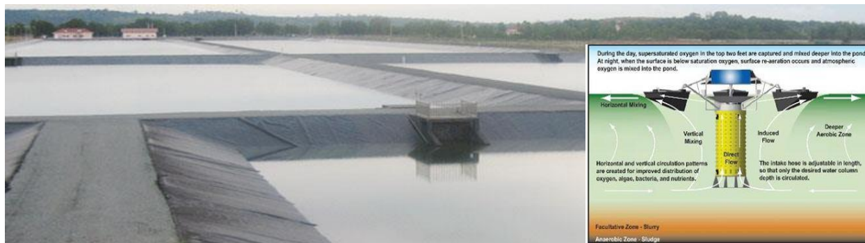
Figure 6 Existing WWTP and Proposed Solar Aerators
