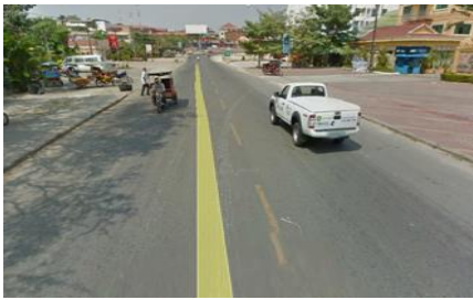
PHOTO 4 RIGHT OF WAY TO INSTALL SEWER PIPE
