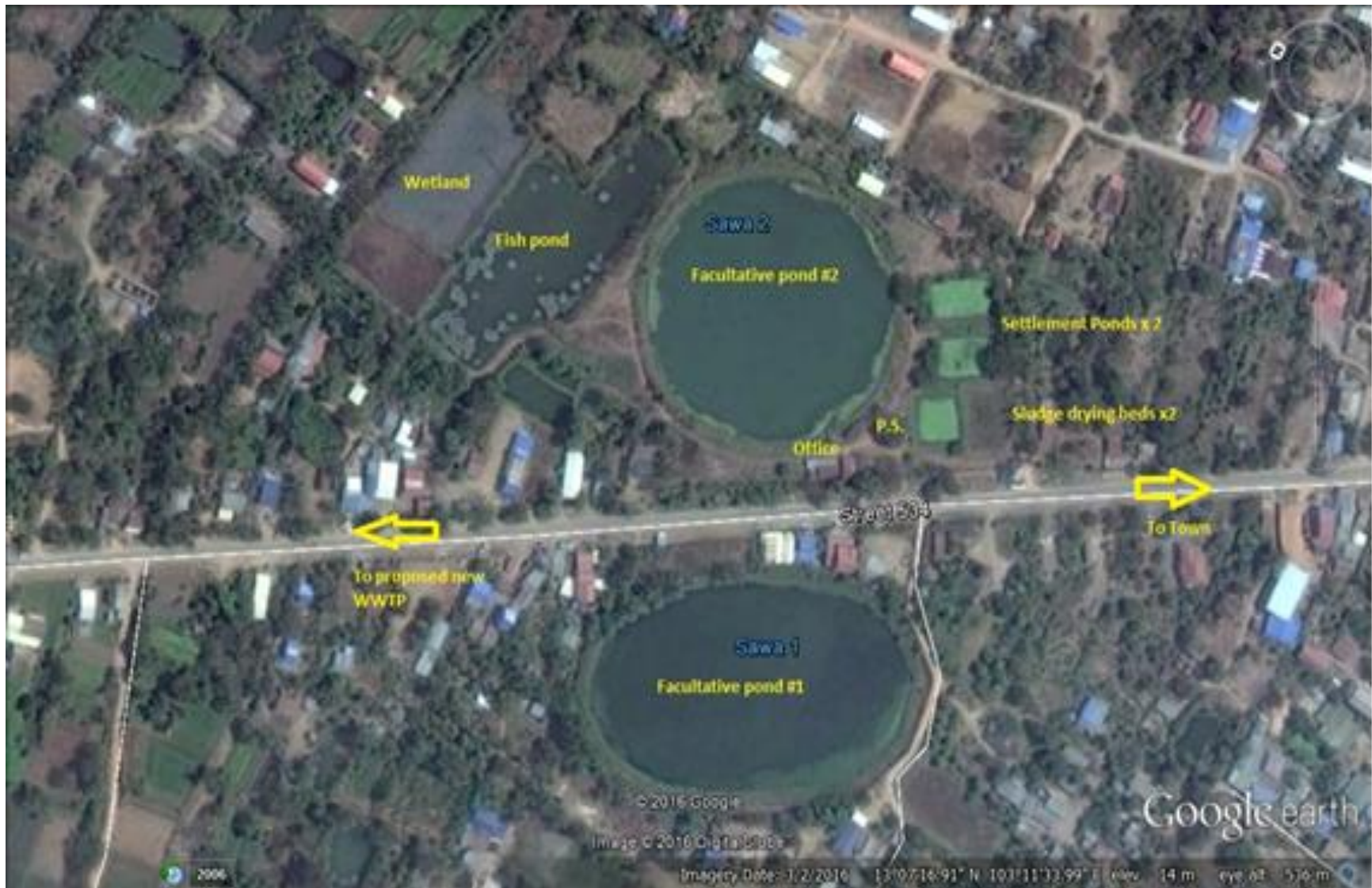
Figure 1: Existing WWTP (constructed in 1994)
