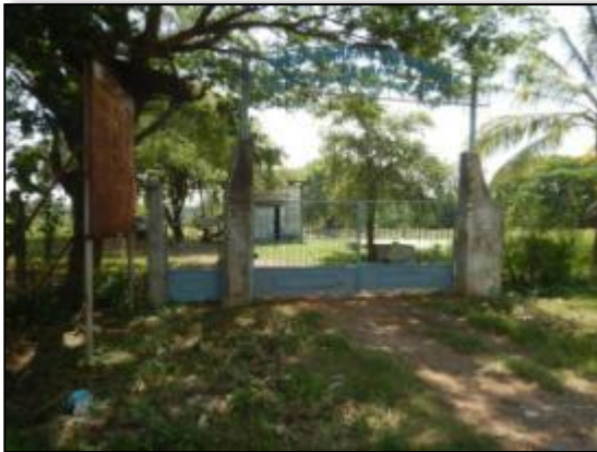
Figure 4-4 Battambang Old WWTP
