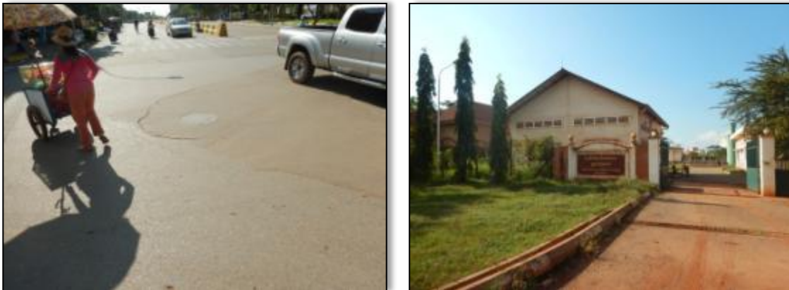
Figure 4-11 Trunk Sewer Manhole and Pumping Station
