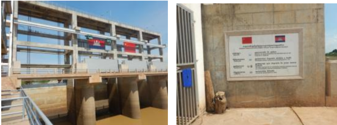
Figure 12-1 Kanghot Irrigation Dam upstream of Off-take Point
