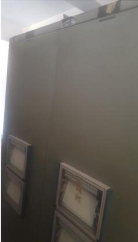
Existing Fault Recorder reported out of order to be replaced
