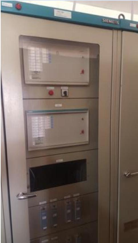
Existing Fault Recorder report out of order to be replaced
