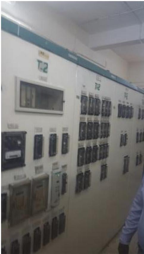
Existing Over Voltage Relay to be replaced
