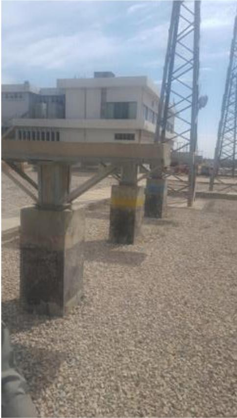
Foundation for new 132kv PT Installation
