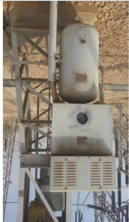
**220 kv Circuit Breakers to be replaced**
