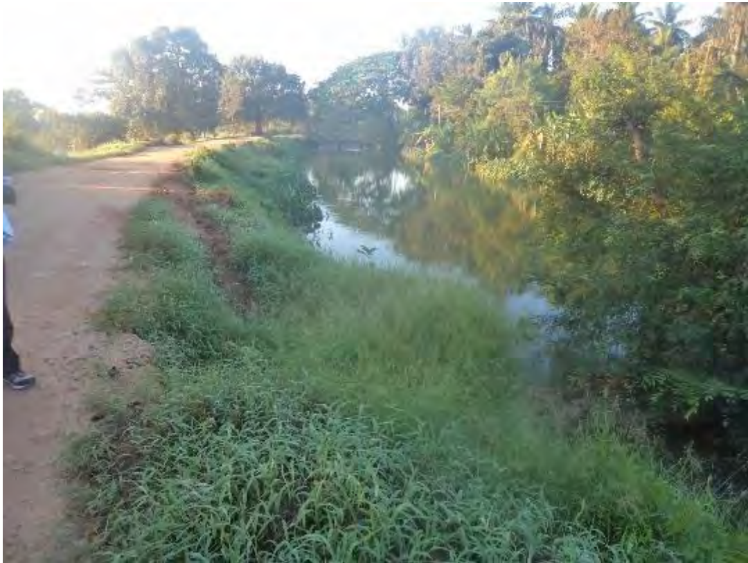
Minipe left bank canal along with the access road.
