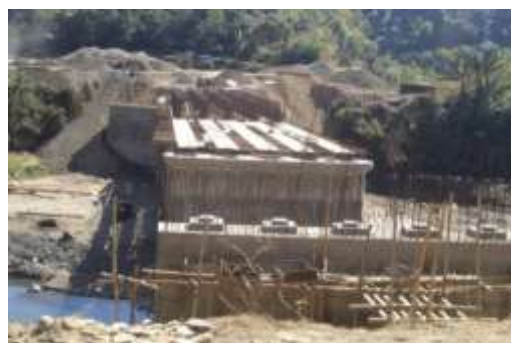
Under construction Bridge at Km 72+450 over Irang River
