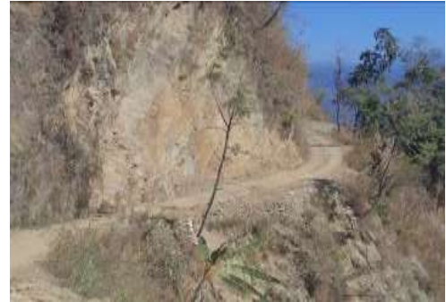
Image 8: Landslide Prone Location along Tamenglong-Bhalok road
