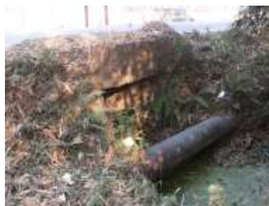
Existing Water Pipe line parallel to project Road
