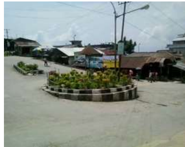
Project end Point at Km 103+00 near Tamenglong
