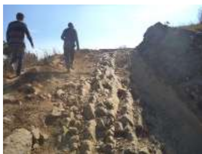
Steep gradient with exposed rock of existing road
