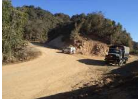
Existing Junction with Senapathi Road at 98+000
