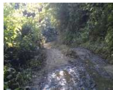
Hill side stream water crossing over existing mud road in absence of drainage
