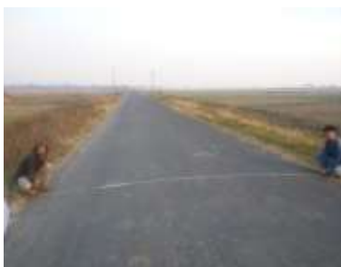
Project Road between Imphal and Kangchup
