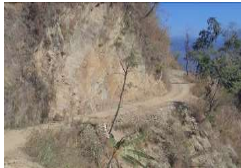
Image 8: Landslide Prone Location along Tamenglong-Bhalok road
