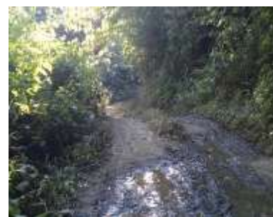
Hill side stream water crossing over existing mud road in absence of drainage
