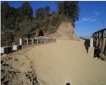
Bridge near Tamenglong
