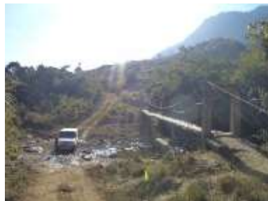
Bailey bridge near Bakuwa over Iring River
