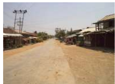
Project road near Kangchup at Km 12
