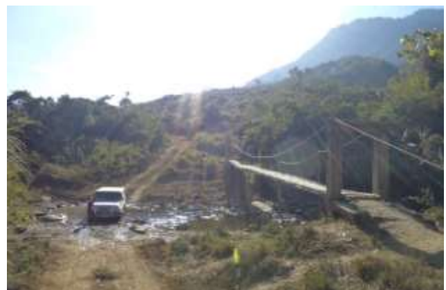
Image 3: Iring River at km 51+900 on Project Riad in hill section
