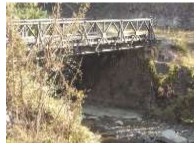
Single Span Steel Bridge over Iring river near Khubu Khulen village
