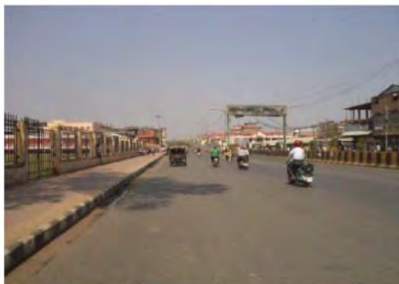
Existing Fly Over approach at Km 0+500
