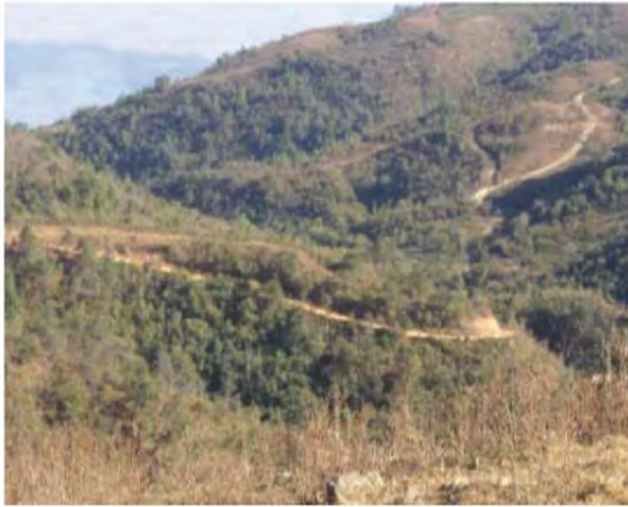
Existing track at km 81 near Warangba Village
