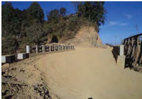
Bridge at Km 108+680 near Tamenglong
