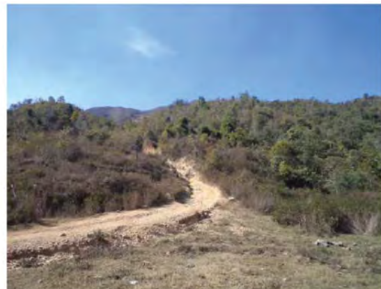
Existing track near Km 40
