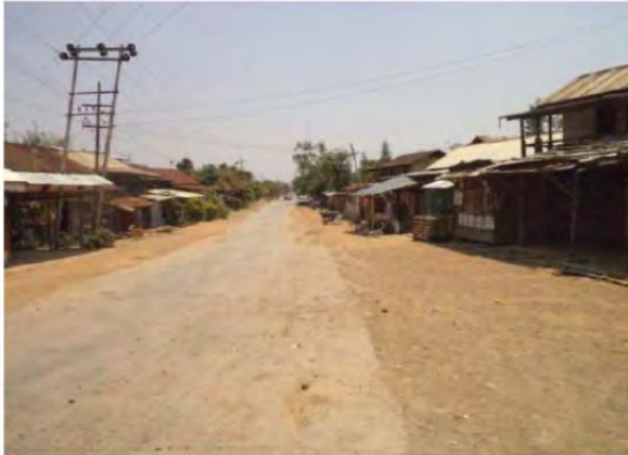
Project road near Kangchup at Km 15
