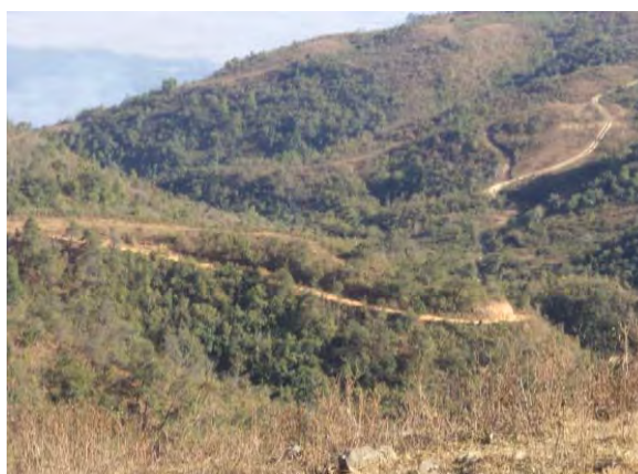
Image 2: Typical Terrain along the Kanchup - Tamenglong Section of Project Road
