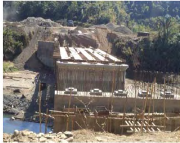
Under construction Bridge at Km 81+075 over Irang River
