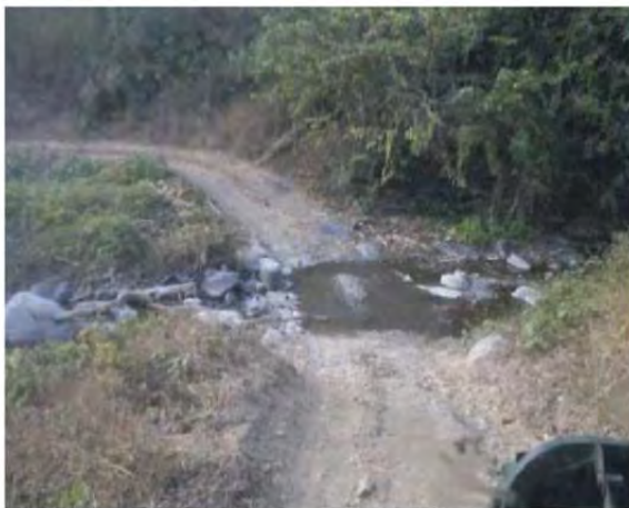
River Duiga at km 85+659
