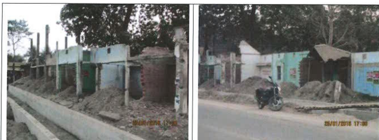
Figure 6: Demolished Structures in AH-48
