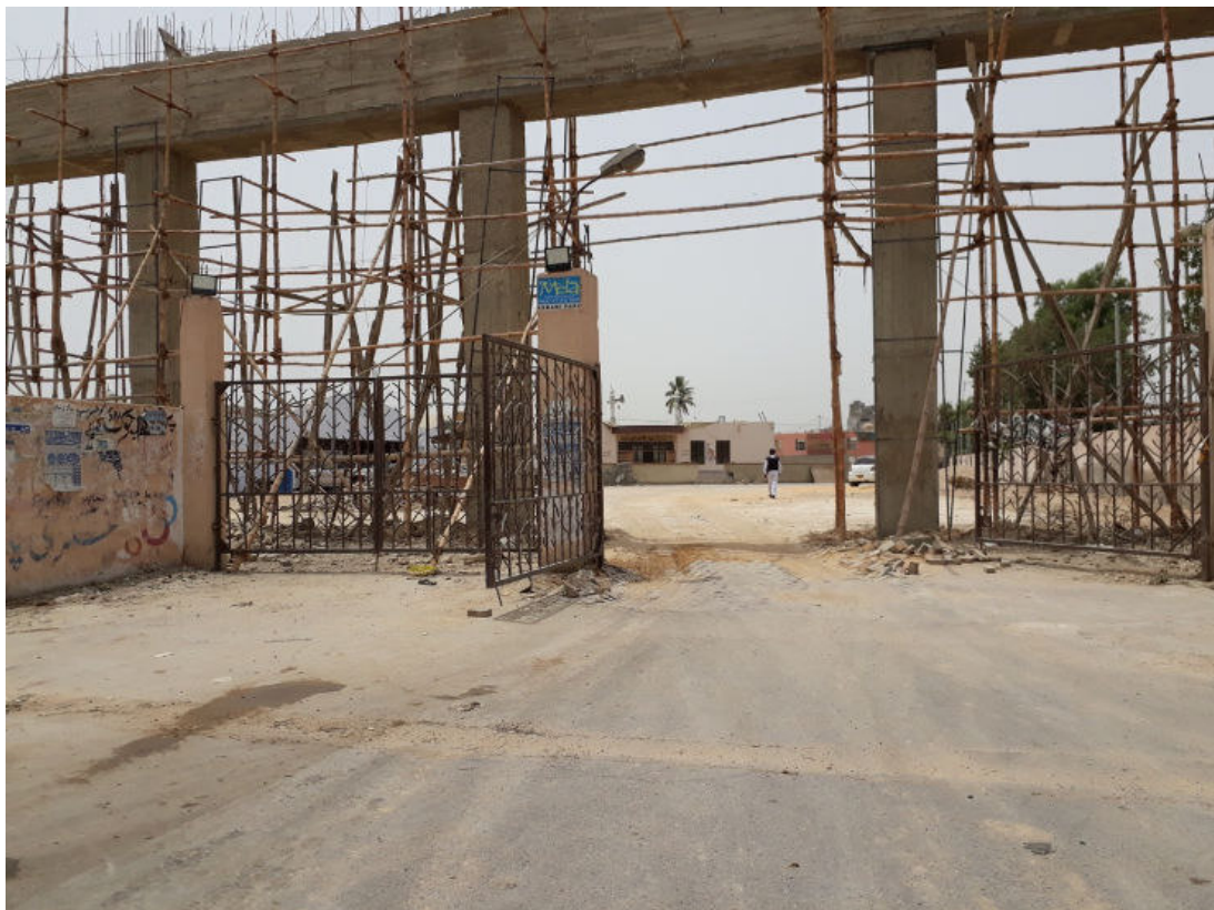
Figure 6-3: Under renovation Askari park (5.00- 12.00 midnight)
