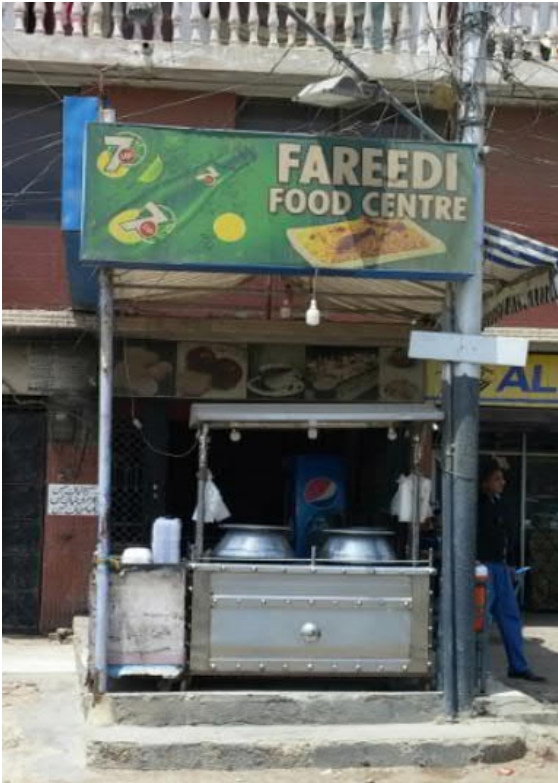
Figure 7: Semi-permanent (poles with marketing sign) and permanent structure (concrete flooring and step) extending into the ROW
