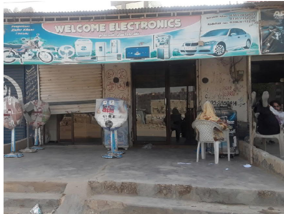
Figure 8: Permanent structure in form of concrete floors, stairs and small boundary extending into the ROW
