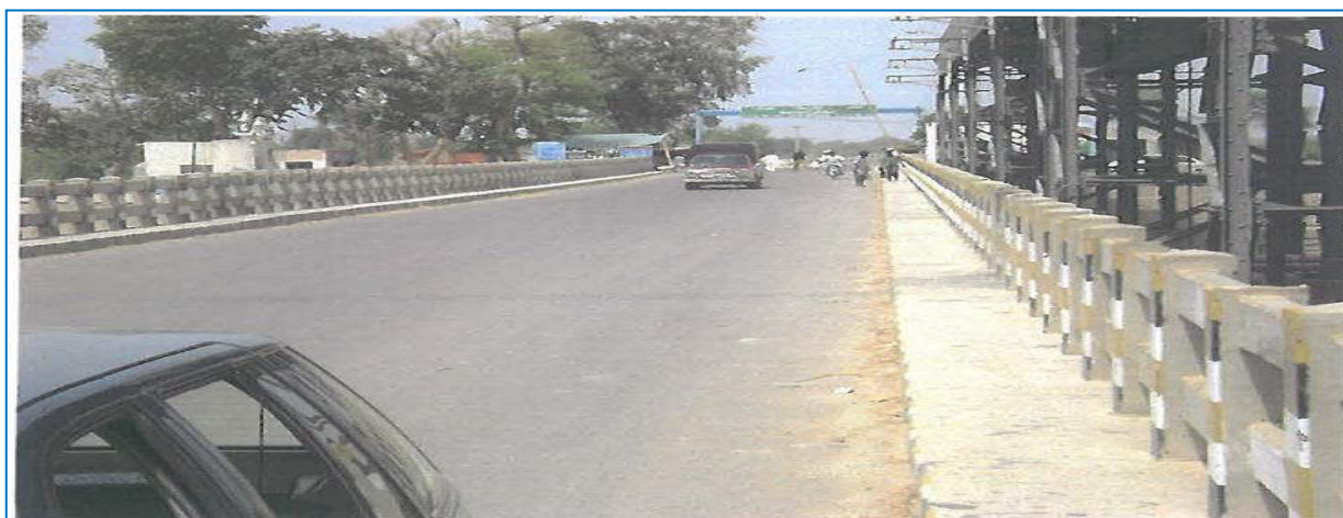
Plate 1.3: Road Bridge on Islam Barrage Main Weir
