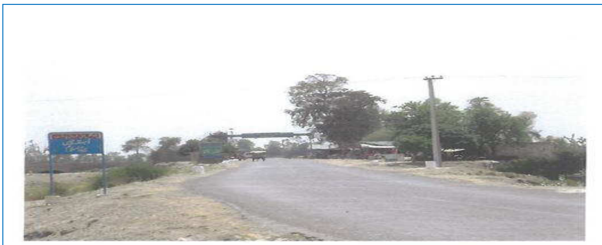
Plate 1.1: Approaching Islam Headworks from Ludden
