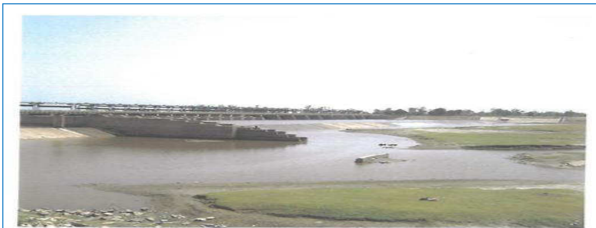
Plate 1.4: Islam Barrage Main Weir and Subsidiary Weir
