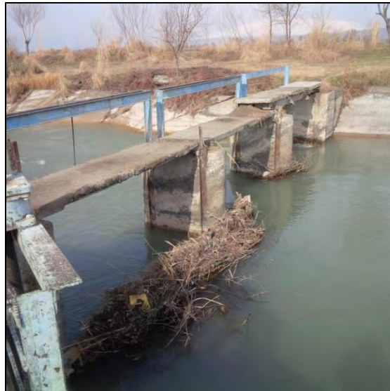
Figure 10: Heavily Damaged Control Gate Structure
