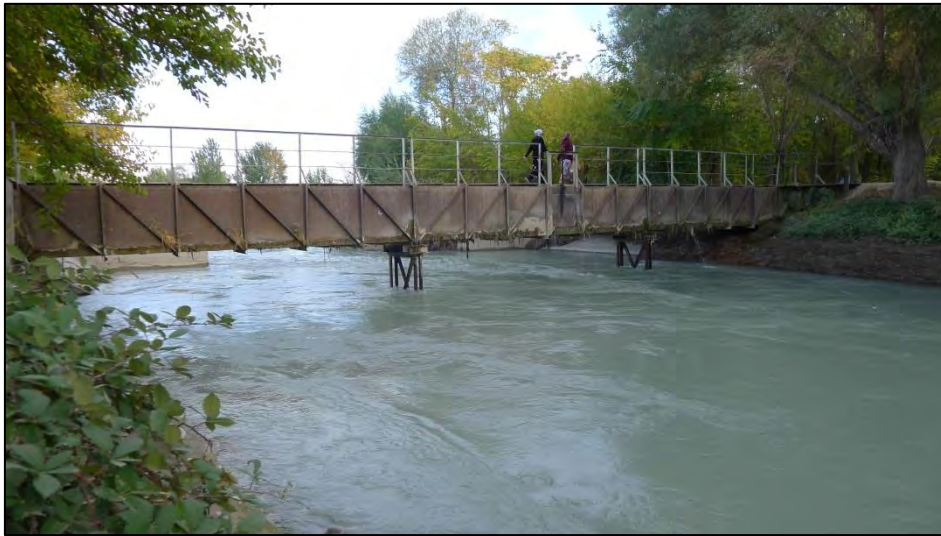
Figure 9: CIS Main Channel, with Aqueduct
