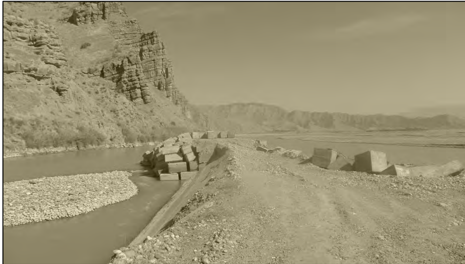
Figure 7: CIS intake. Note Flood Protection Works
