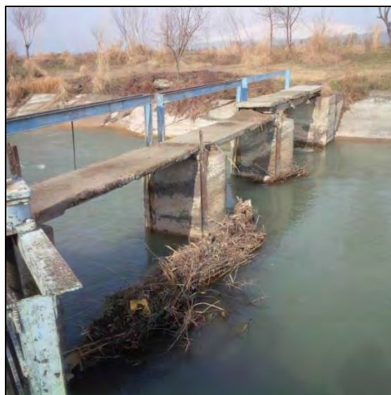
Figure 10: Heavily Damaged Control Gate Structure
