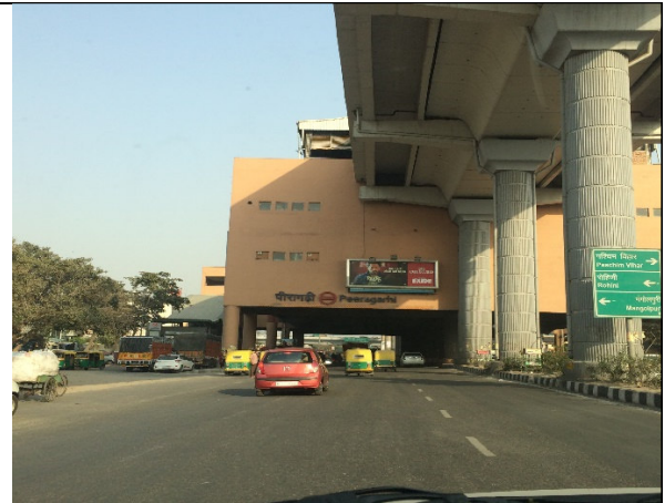
Line 20 Transmission route leading to Mongolpuri, Peeragarhi, and Paschim Vihar area.
