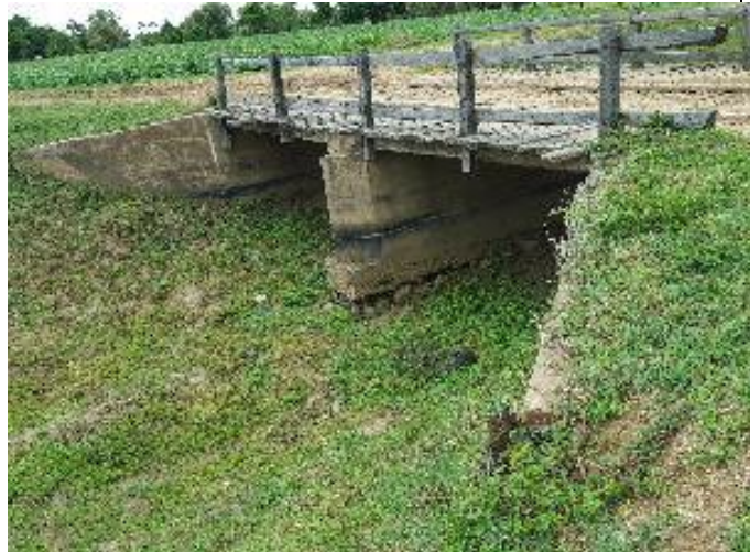
CM Bridge (RD 7373')
