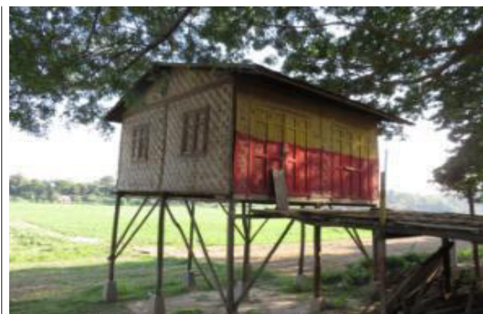
Figure 3 Affected structure in WWTP site. (November 2014)
