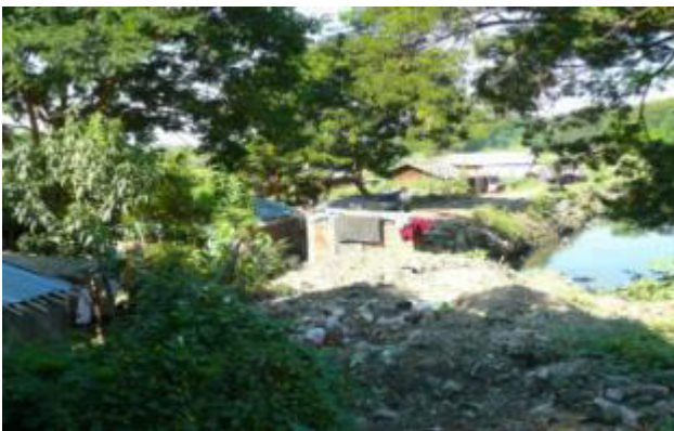
At MDCDC existing pumping station
