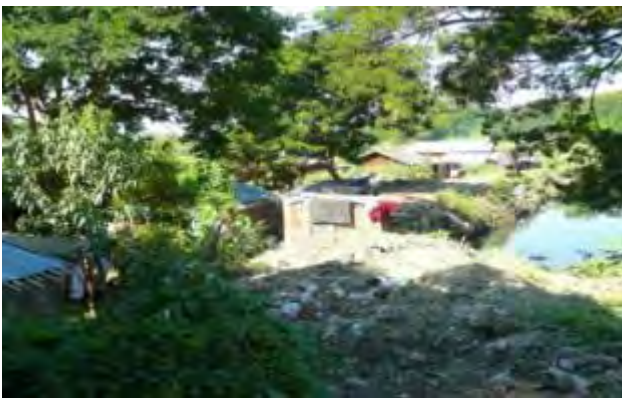
At MDCDC existing pumping station
