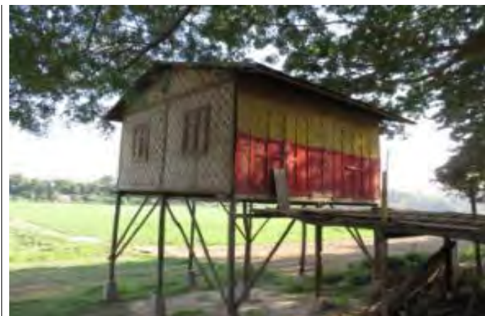
Figure 3 Affected structure in WWTP site. (November 2014)
