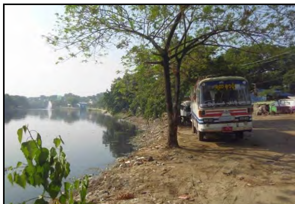
GENERAL ASPECT OF THE WEST SHORE ALONG WHICH INTERCEPTOR WILL BE LAID
