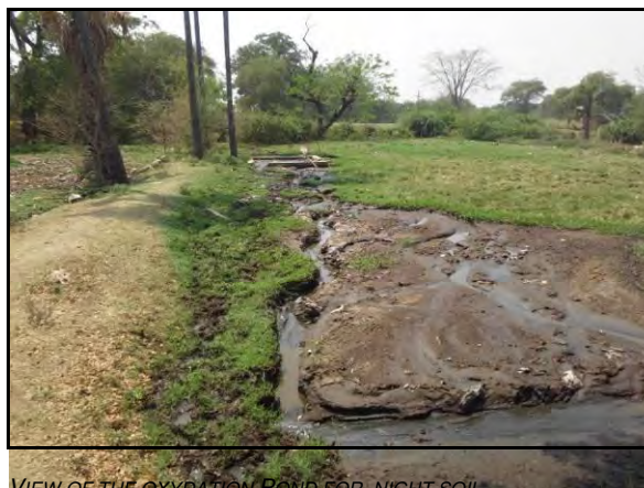
VIEW OF THE OXYDATION POND FOR NIGHT SOIL
