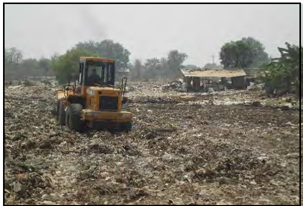
BULDOZER OPERATING ON SOUTH LANDFILL
