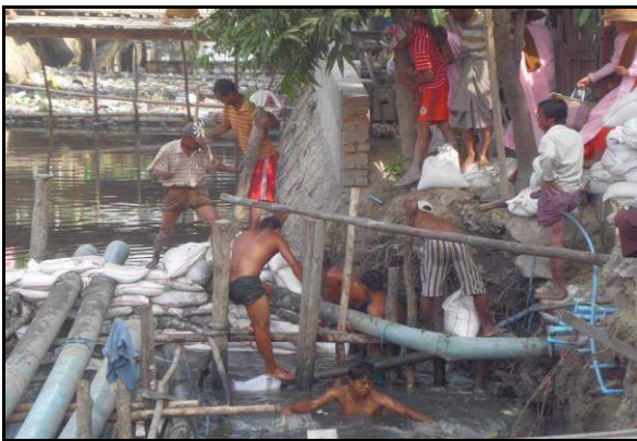
ABSENCE OF ANY BASIC OCCUPATIONAL HEALTH AND SAFETY MEASURES ON THIS CONSTRUCTION SITE ALONG SHWE TA CHAUNG CANAL
