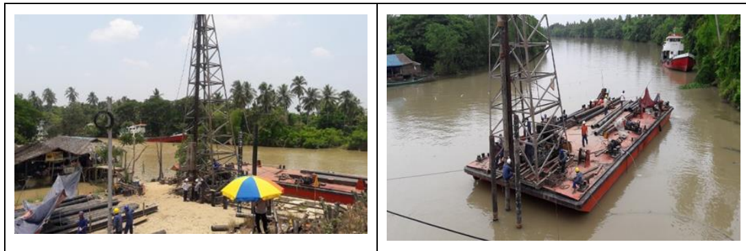
Figure 11. Installation of the piers on the river bank and in-the-water for the temporary Oo Yin Chaung Bridge
