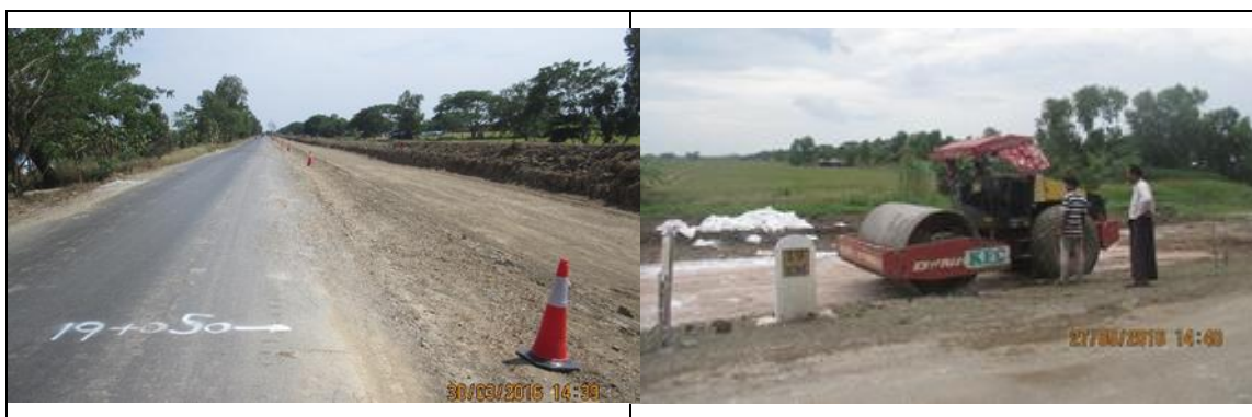
Figure 4. Excavation of unsuitable materials Km 19 to 22 and lime stabilization
