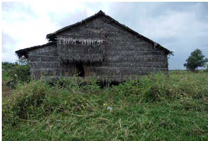
Photo 3: U Moe Swe's Secondary Structure made of Bamboo and Nipa (side view)
