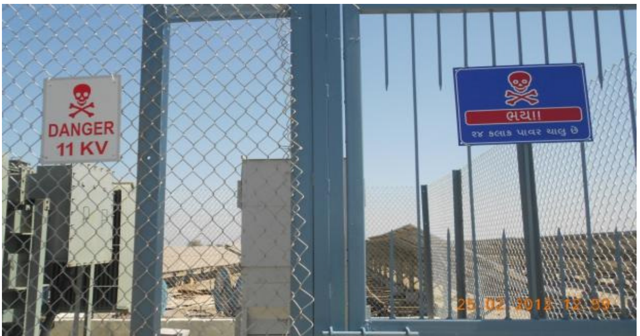
Photograph showing the display of restricted area/danger signage for the workers near the electrical area (Also displayed in local language)
