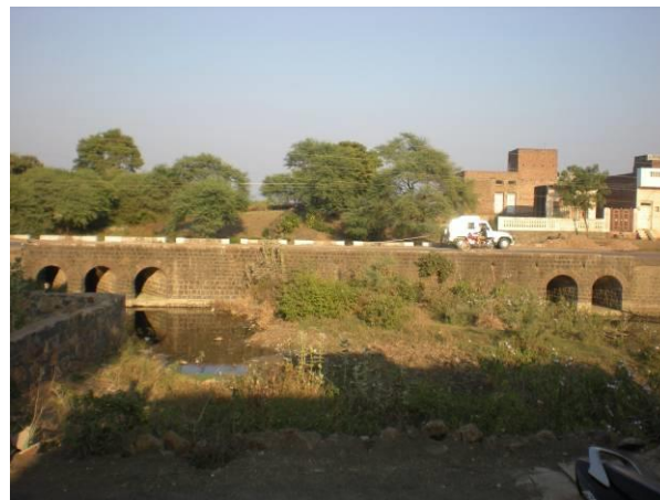
Photo 2.4: Causeway at Km 75+990 (5x4.10x2.80)
