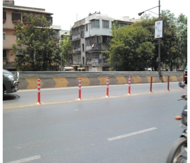
Delineators/ guard poles on flyover for lane separation.
