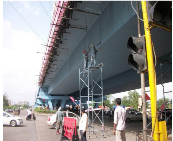
Barricade separating work & traffic area
