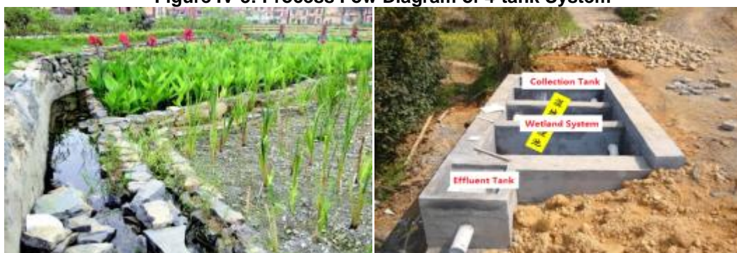
Figure IV-4: Typical 4-tank System
