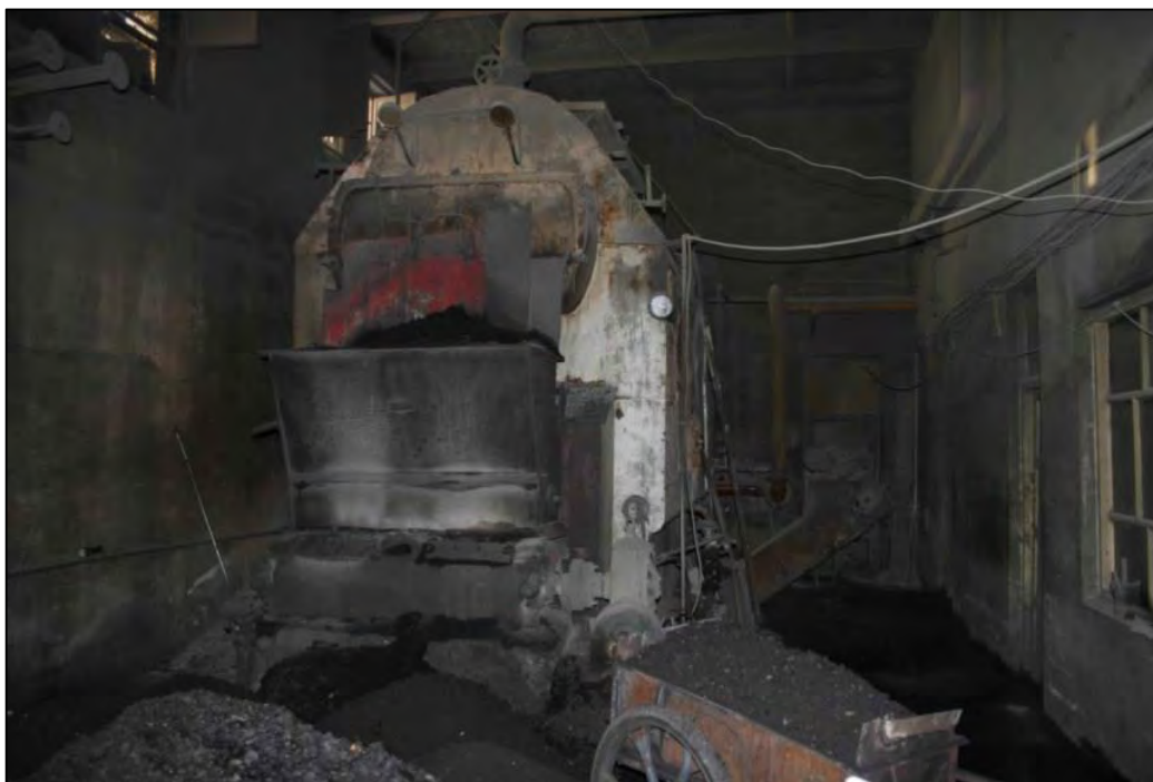
Figure 4: Existing low efficiency coal-fired boiler in Jinqiao heating zone. The boiler will be decommissioned and dismantled once the Project becomes operational.
