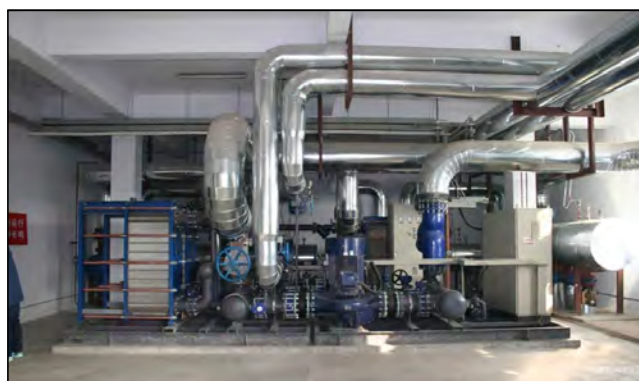
Figure 12: Interior of two-unit automated district HES built in 2011.
