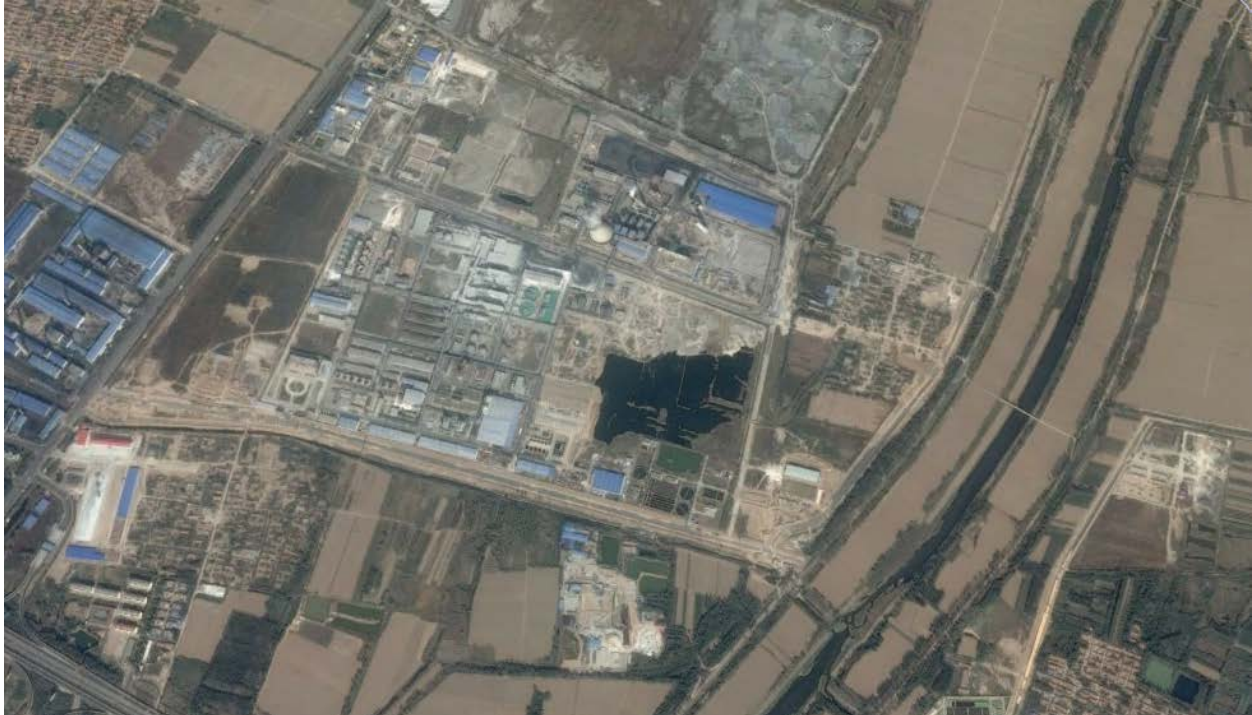
Figure 2: Closer View of the Dezhou Shihua Chemical Plant
