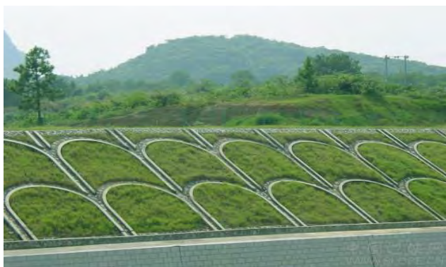
Figure V-4: Arch Concrete-Framed Vegetation Slope Protection (Design III)
