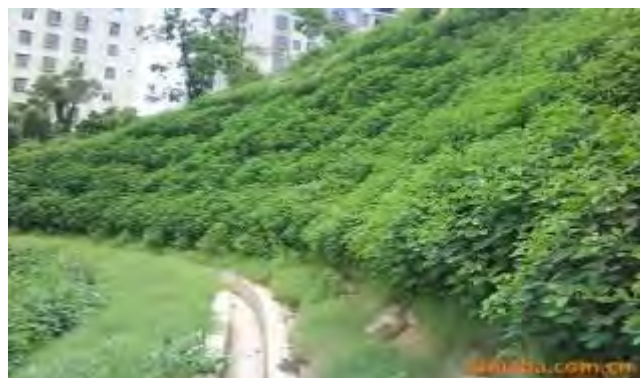
Figure V-5: Natural Vegetation Slope Protection with Intercepting Drain (Design I)
