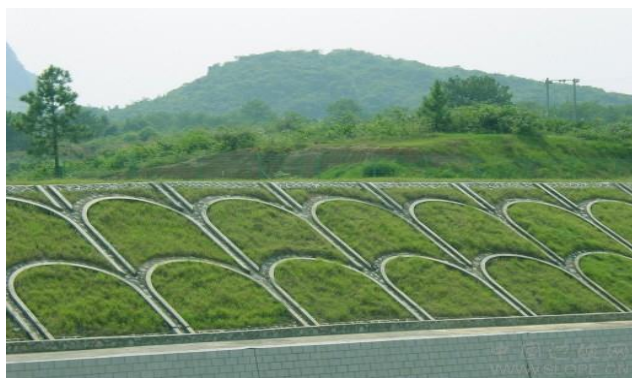
Figure V-4: Arch Concrete-Framed Vegetation Slope Protection (Design III)
