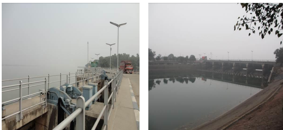
Figure 6.30: Head Regulator Rasul Qadirabad Link canal at the Rasul Barrage
