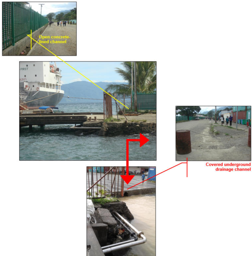
Figure 3.1: Location of the Drainage Discharge Points at the Seawall and Current Backflow During High Tide Level
