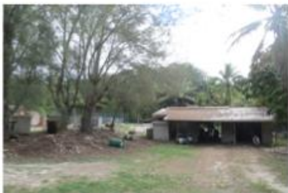
Existing power house in Mauke Island to be relocated to proposed solar power plant
