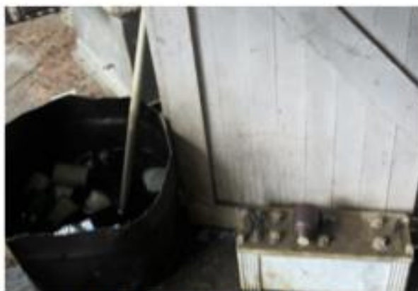
Existing practices for used oil and battery management in Mauke powerhouse need immediate attention
