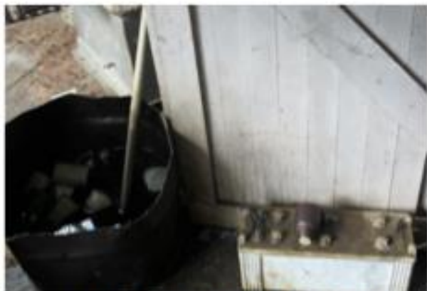
Existing practices for used oil and battery management in Mauke powerhouse need immediate attention
