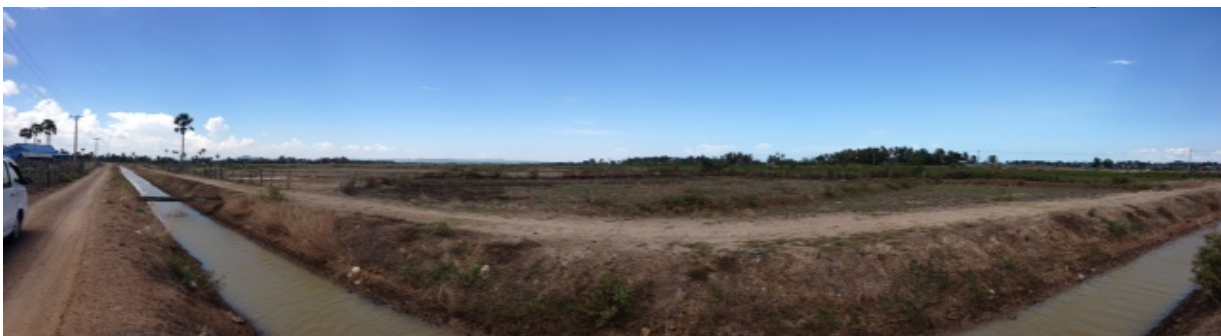
Figure 1: The WWTP site
