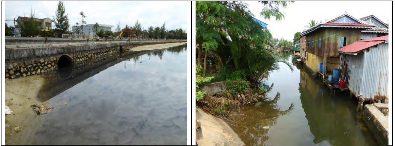
Figure 19. Example town drain outfall to Teuk Chhou river, and WW canal
