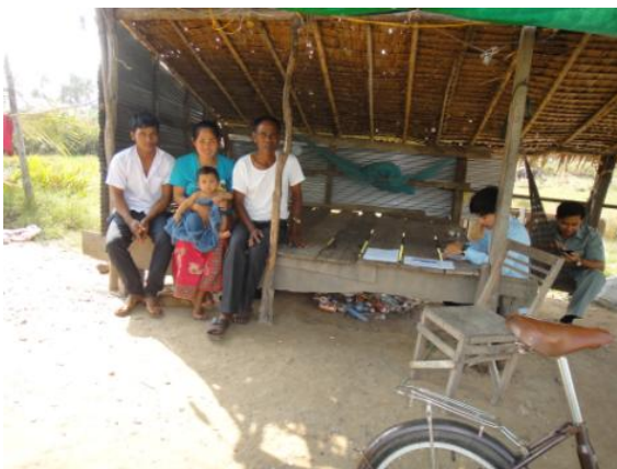
Temporary shelter made of leaf roof, wood frame wood sleeping space size: 3m x 3m (45$)
