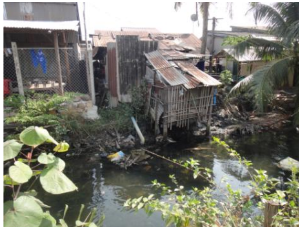
Along the canal near bridge on road to Kep (45$) Pigpen made of wood wall and zinc roof wood floor size:1.5m x 1.5m
