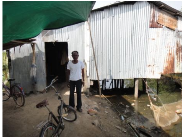
Small house made of zinc wall and roof Wood frame and sleeping space 5m x 4m Along the canal from Chak Pond (250$)
