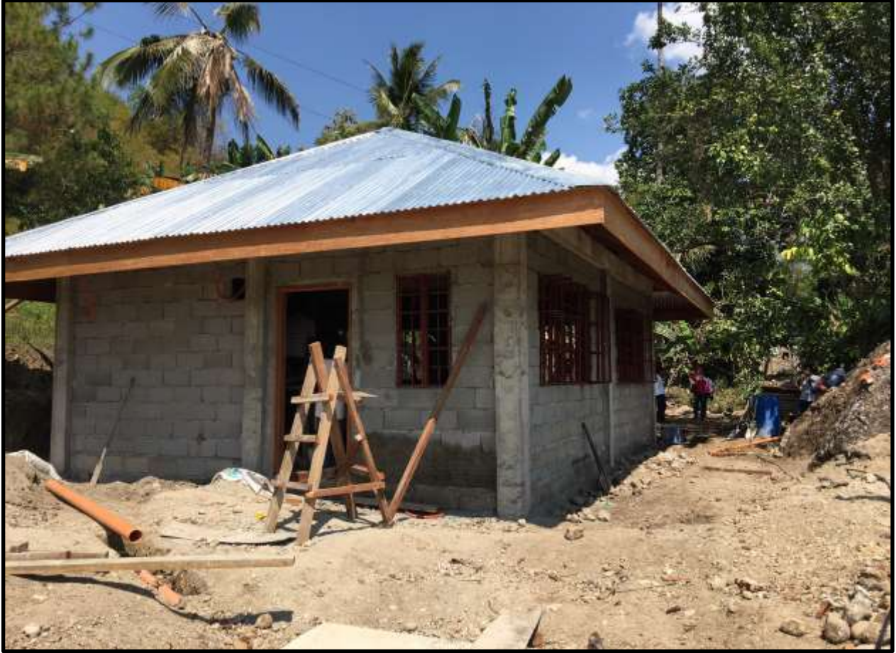
On-going Construction of Day Care Center in Barangay Cuba, Kapangan, Benguet
