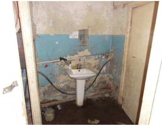
Photo 4-11: If washing facilities exist, they are badly maintained
