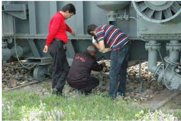
Photo 4-18: Oil sampling from autotransformers
