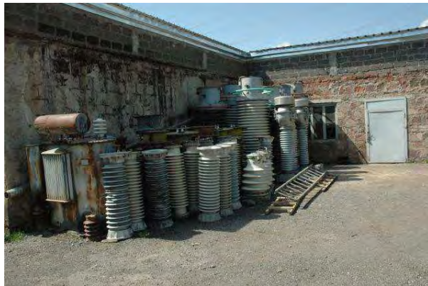
Photo 4-15: Ceramic waste stored at a substation site
