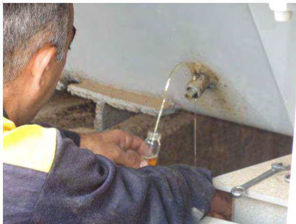
Photo 4-19: Oil sampling from autotransformers
