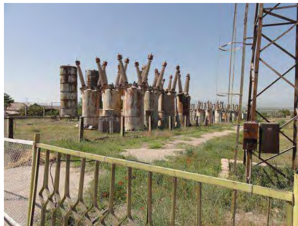
Photo 4-13: Old circuit breakers stored at substation site sometimes since decades
