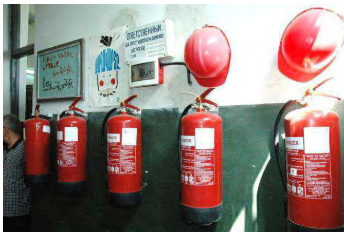
Photo 4-7: Sufficient well maintained powder based fire extinguisher were available inside the control buildings of all substations
