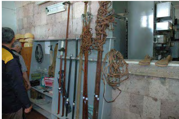
Photo 4-9: Basic safety equipment as helmets, gloves, tools for working under high voltage and signs at the substations
