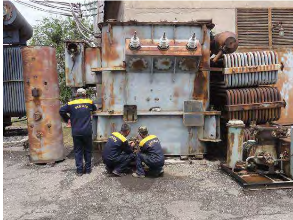
Photo 9-1: Discarded equipment is used for storage of old and/or spare oil. This old equipment is often leaking.
