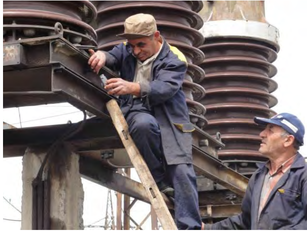
Photo 4-17: Oil sampling from a circuit breaker being cut off
