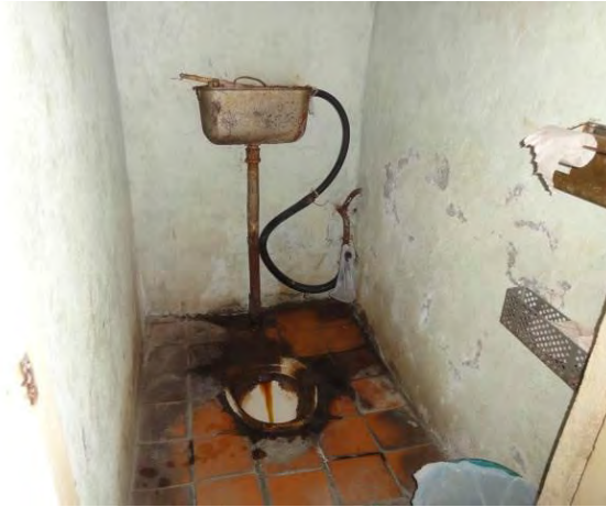
Photo 4-10: Typical toilet at a substation, if existing at all
