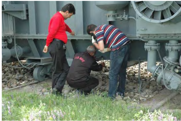
Photo 4-18: Oil sampling from autotransformers
