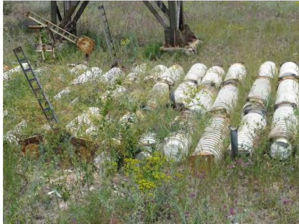
Photo 4-14: Ceramic waste stored at a substation site
