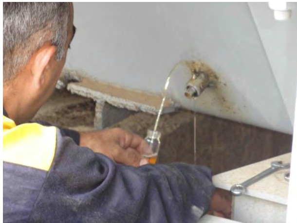
Photo 4-19: Oil sampling from autotransformers
