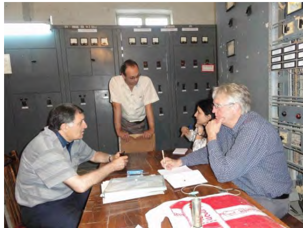
Photo 7-1: Discussion at a substation
