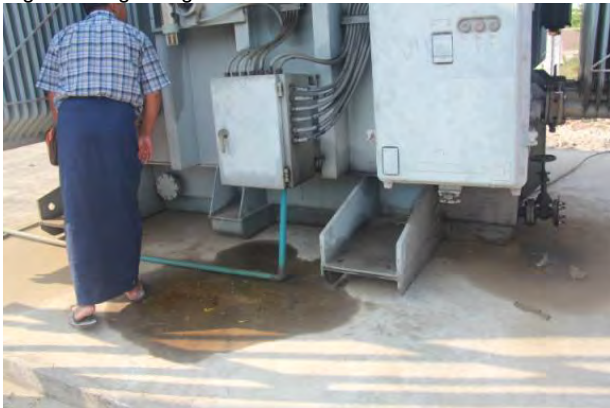
Signs of transformer oil leak on the pavement
