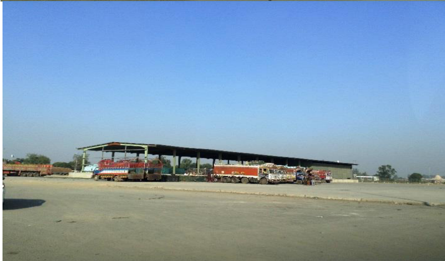
View of existing yard operated by National Logistic Cell, Wagah, Pakistan
